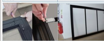
After turning all screws at the four corners. please adjust the junctures of the corners. Installation of inner frames and support Hold the frame tightly with one hand and tighten the screws with the other hand.
